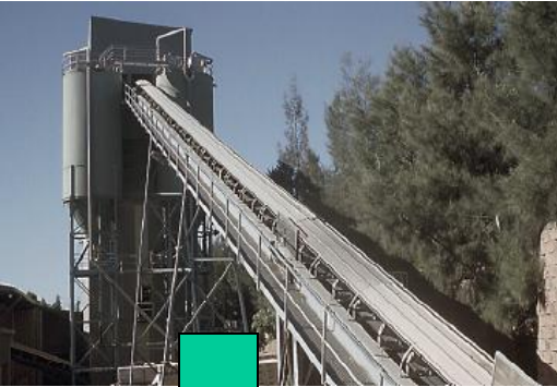
Raw materials delivery, storage & retrieval
