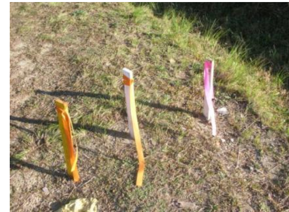
Corner or Offset Pegs with Marker Pegs
