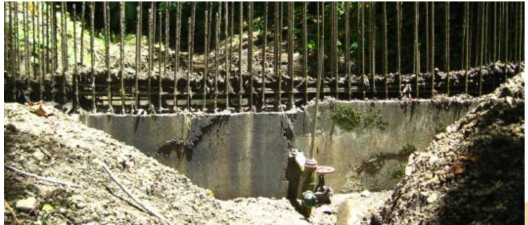
Vertical reinforcement for future extension
