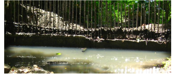
Vertical reinforcement for future extension
