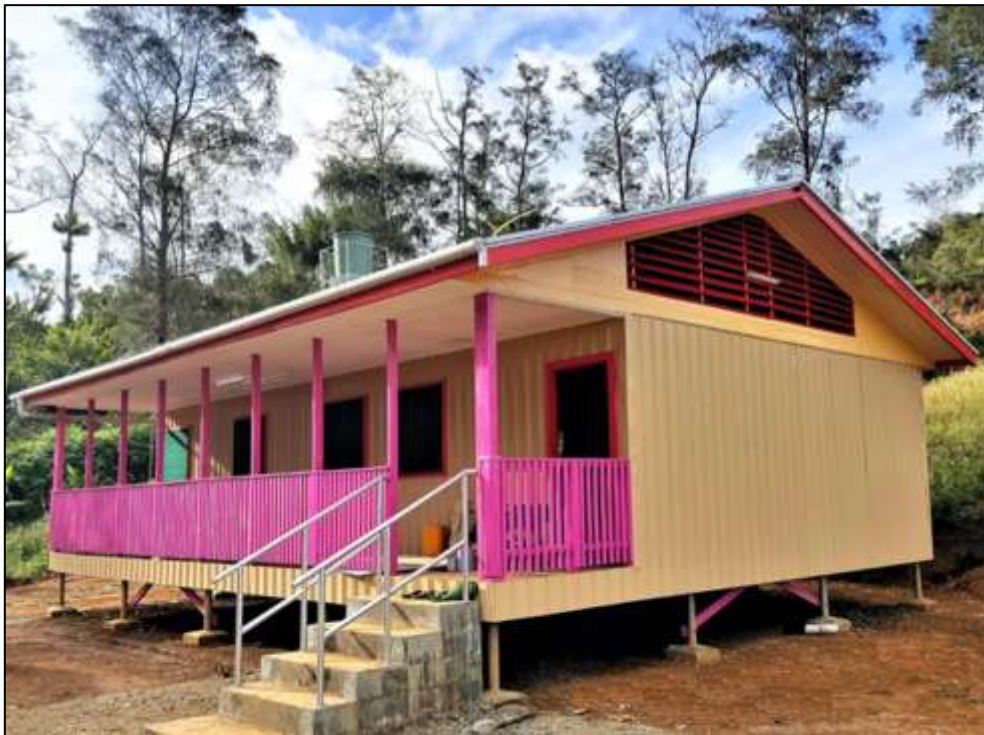
Kopeng Community Health Building in the Papua New Guinea Western Highlands Province using the Partner Housing Australasia DANCER Building System
